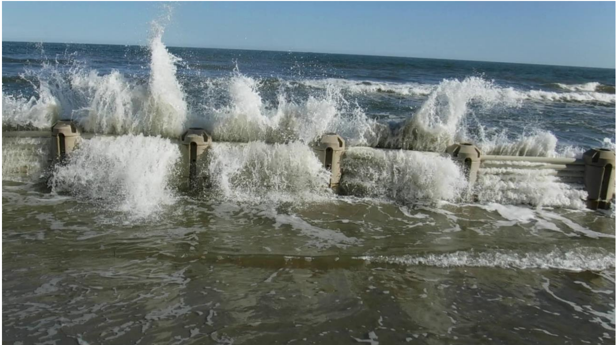
Figure 4-105. Example of wave breaking and water jetting through WDS at BE
