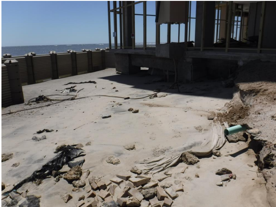
Figure 4-75. April 18 photograph from east side of OC looking south
