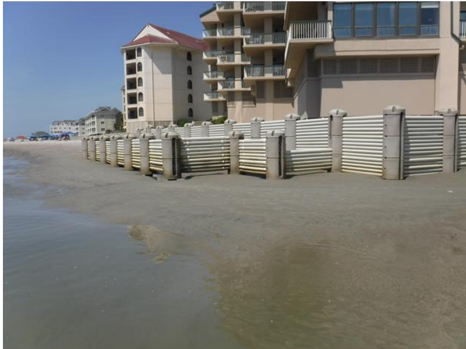
Figure 4-85. July 13 photograph of southeast corner of three-tier WDS section
