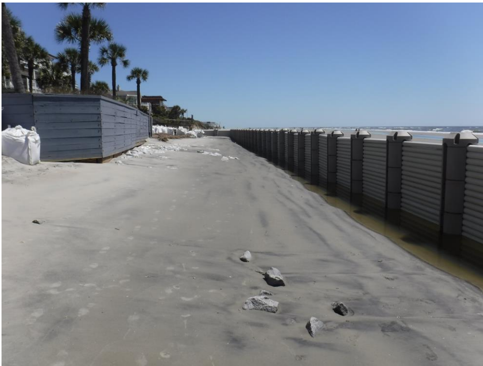
Figure 4-47. April 18 photograph south of the bulkhead looking northeast
