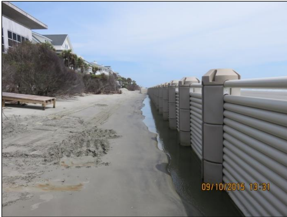
Figure 2-30. WDS at BE in September 2015 following removal of sandbags (source: SCDHEC-OCRM)
