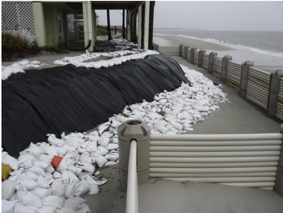
Figure 4-17. May 19 photograph looking northwest in front of lot 52
