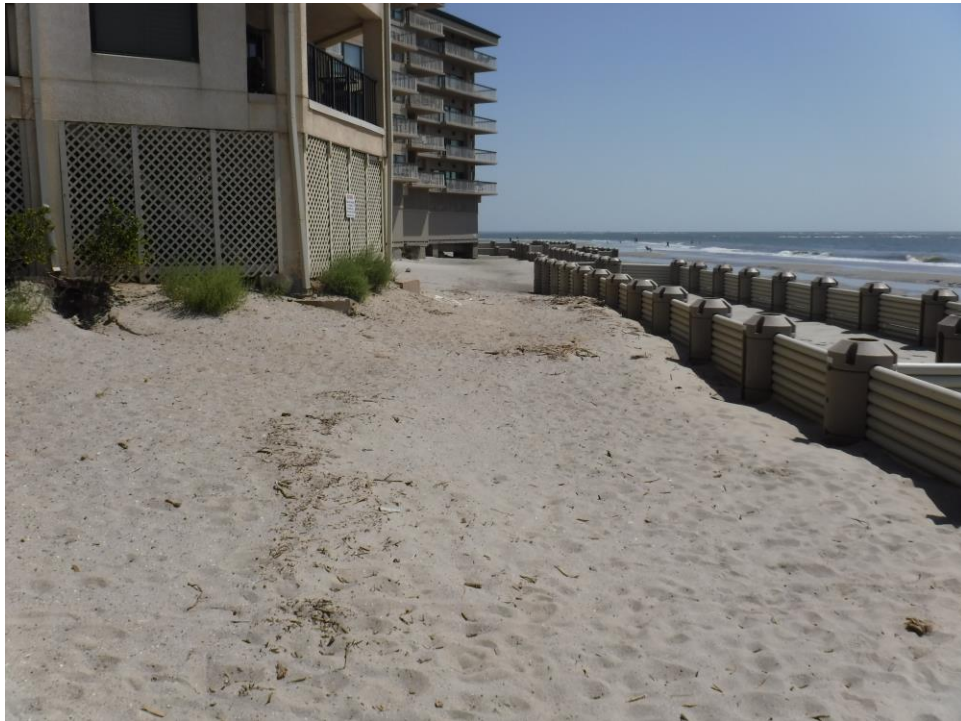
Figure 4-68. July 13 photograph looking east from SV
