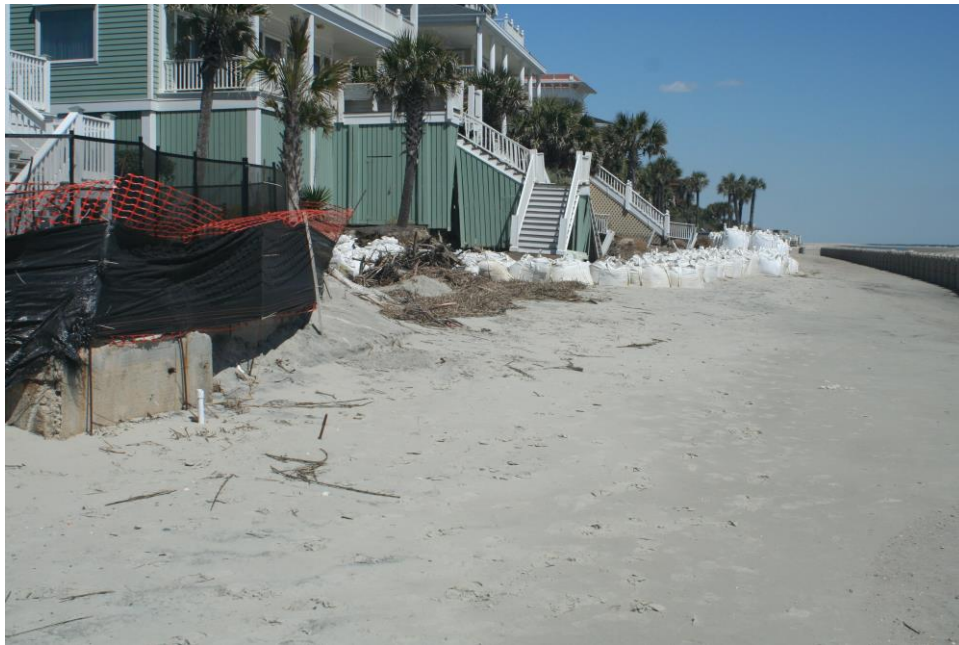
Figure 4-42. March 21 photograph from the community access point looking northeast
