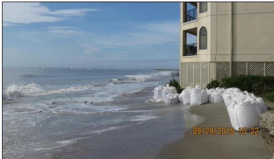
Figure 2-15. Sand bags in front of Seascape Villas prior to 2015 WDS installation (source: SCDHEC-OCRM)
