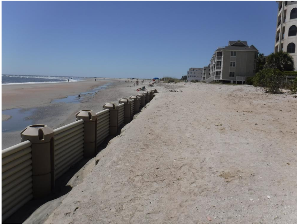
Figure 4-62. April 18 photograph looking past the west end of the WDS
