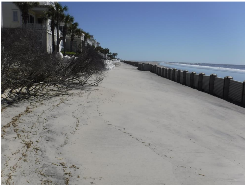
Figure 4-39. April 18 photograph from south end of WDS towards northeast
