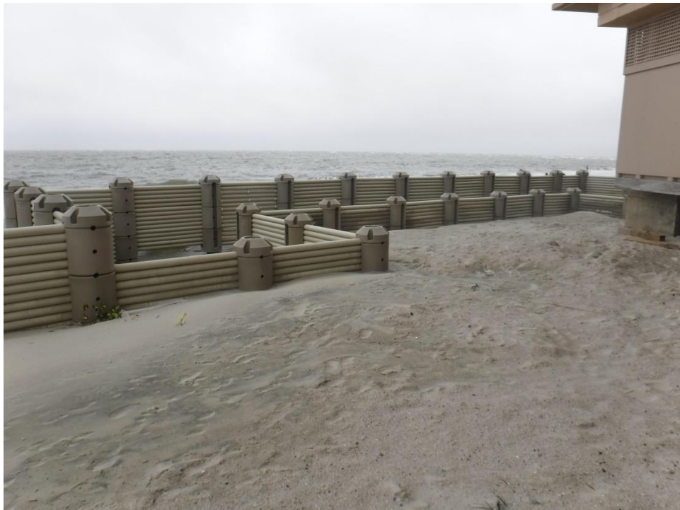
Figure 4-76. May 20 photograph from east side of OC looking south
