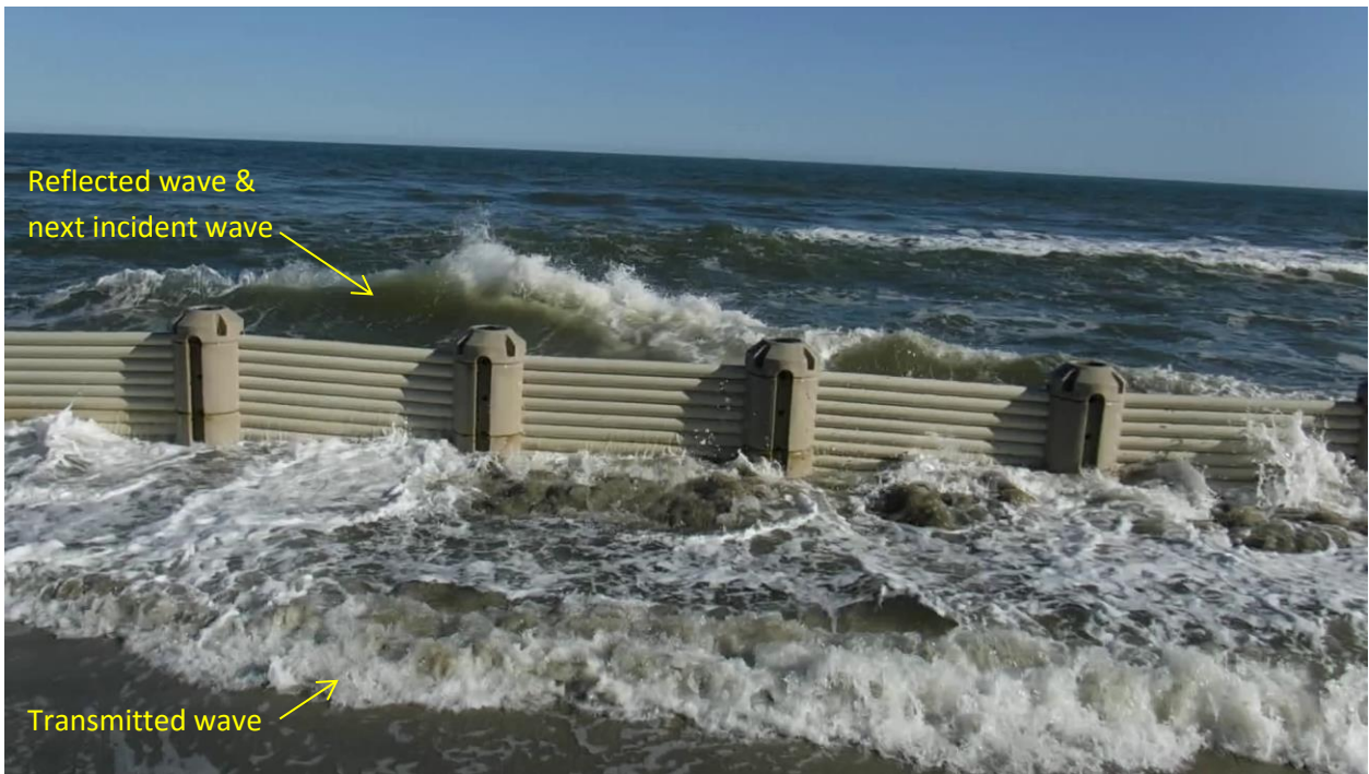
Figure 4-106. Example of transmitted and reflected waves from same incident wave in Figure 4-105
