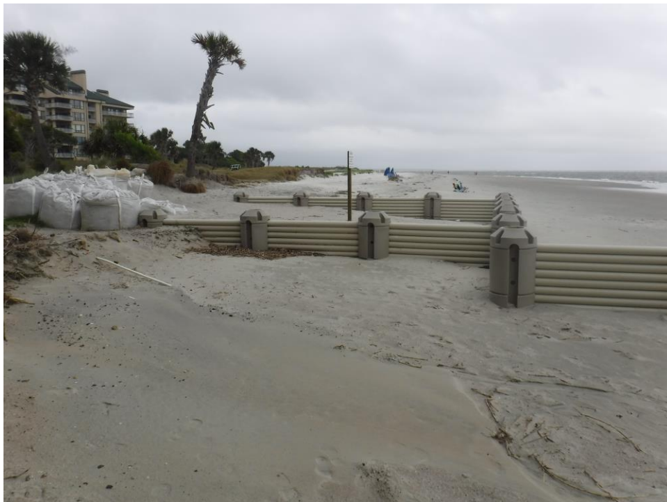
Figure 4-80. May 20 photograph from east side of OC looking east
