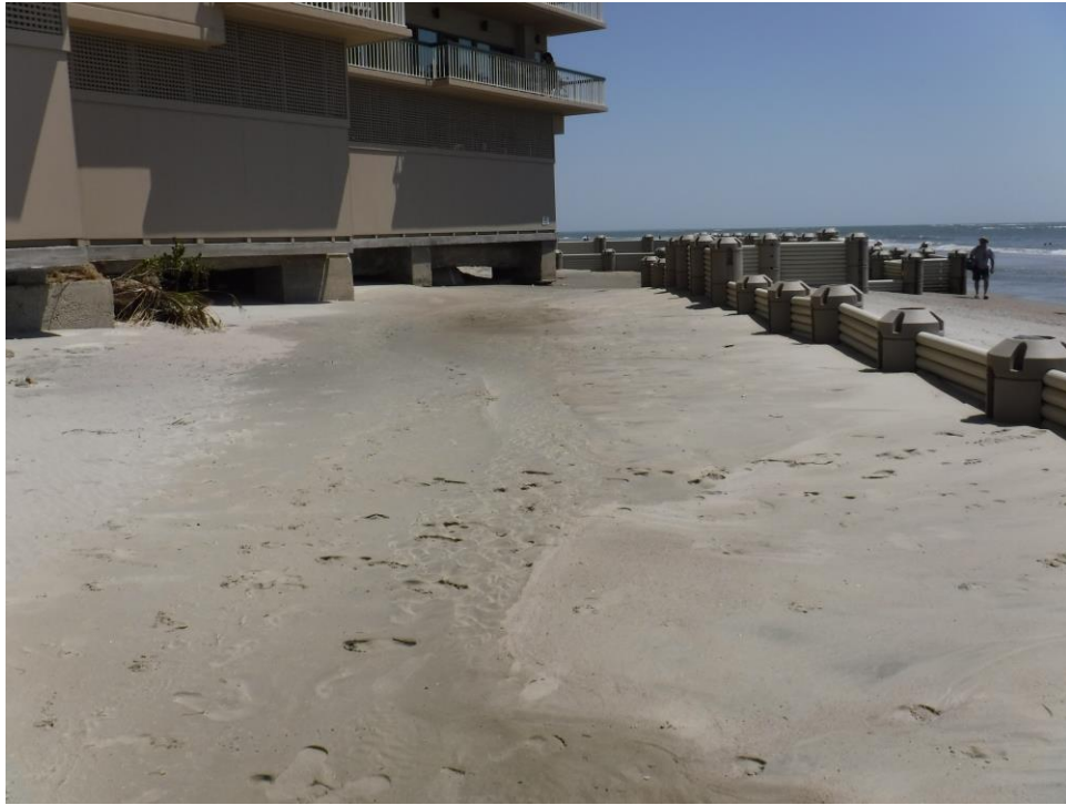
Figure 4-72. July 13 photograph looking east toward OC building
