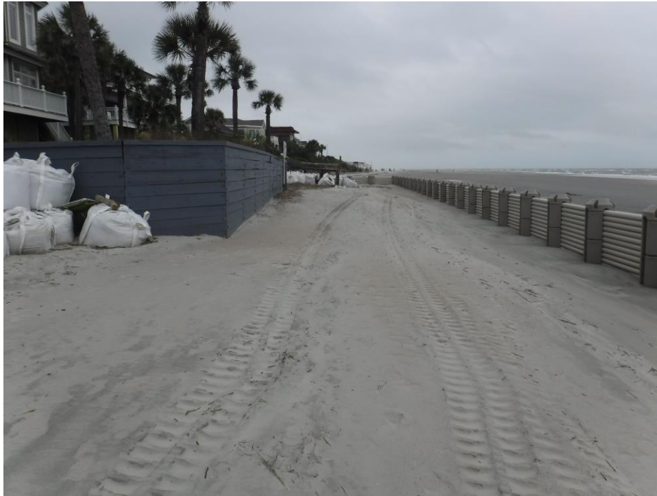
Figure 4-48. May 20 photograph south of the bulkhead looking northeast
