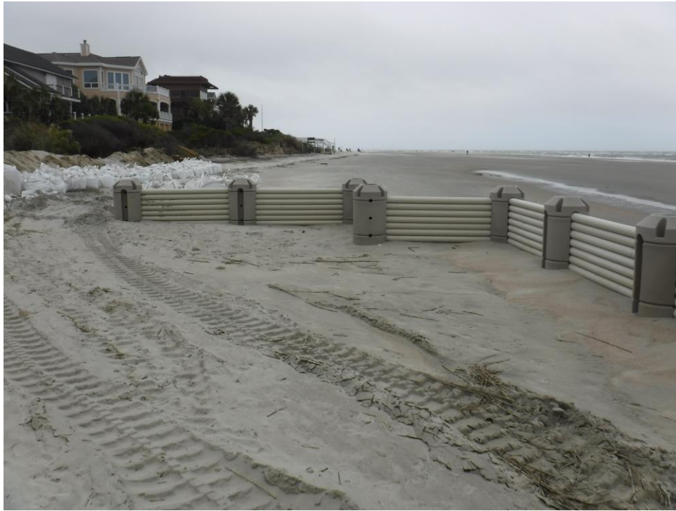
Figure 4-52. May 20 photograph from east end of WDS looking northeast
