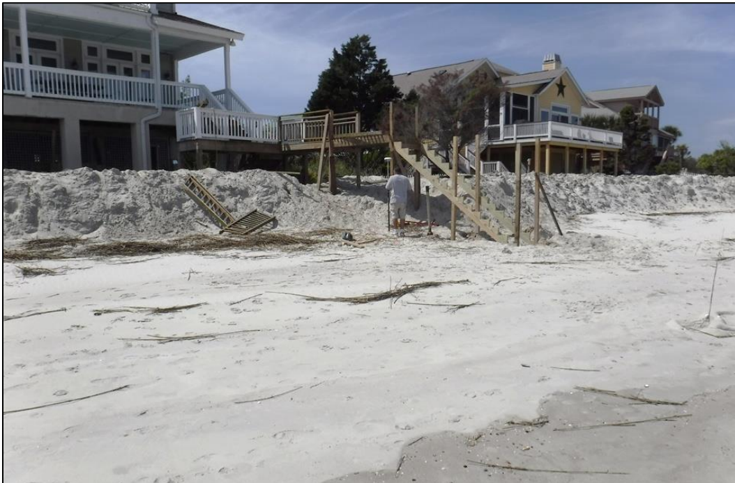
Figure 2-7. Minor renourishment sand placed in dune north of WDS (March 24, 2016)
