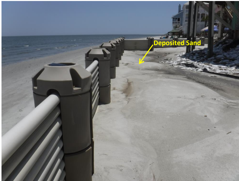
Figure 5-1. Sand passed through WDS at Harbor Island during mild wave conditions (July 14, 2016)
