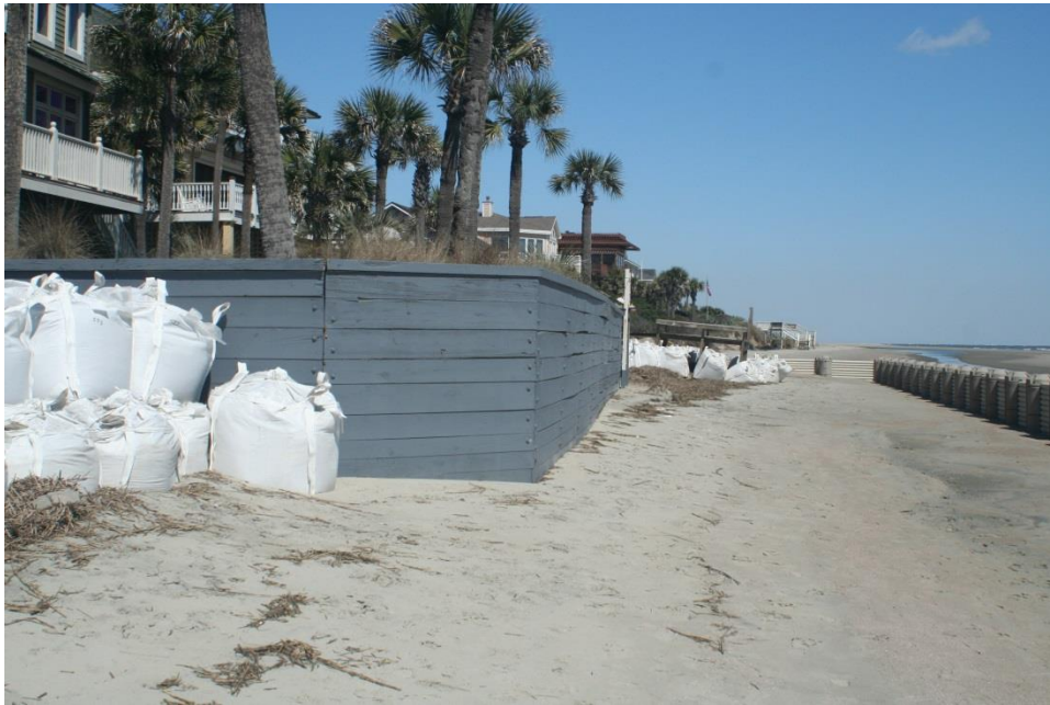
Figure 4-46. March 21 photograph south of the bulkhead looking northeast
