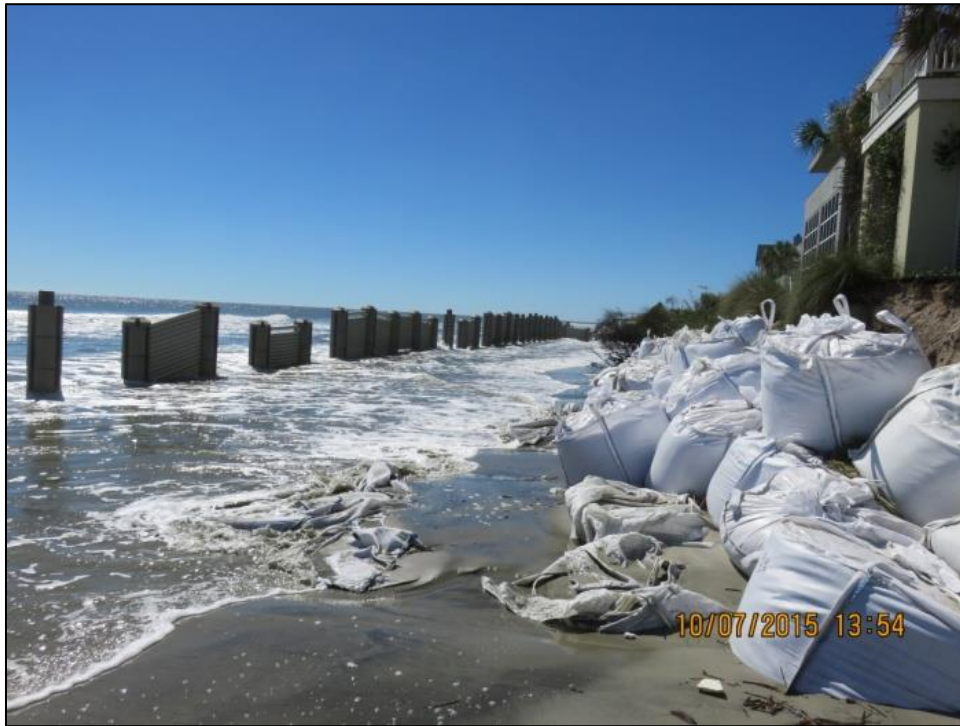
Figure 2-32. WDS at Beachwood East following Hurricane Joaquin; view towards the southwest (source: SCDHEC-OCRM)
