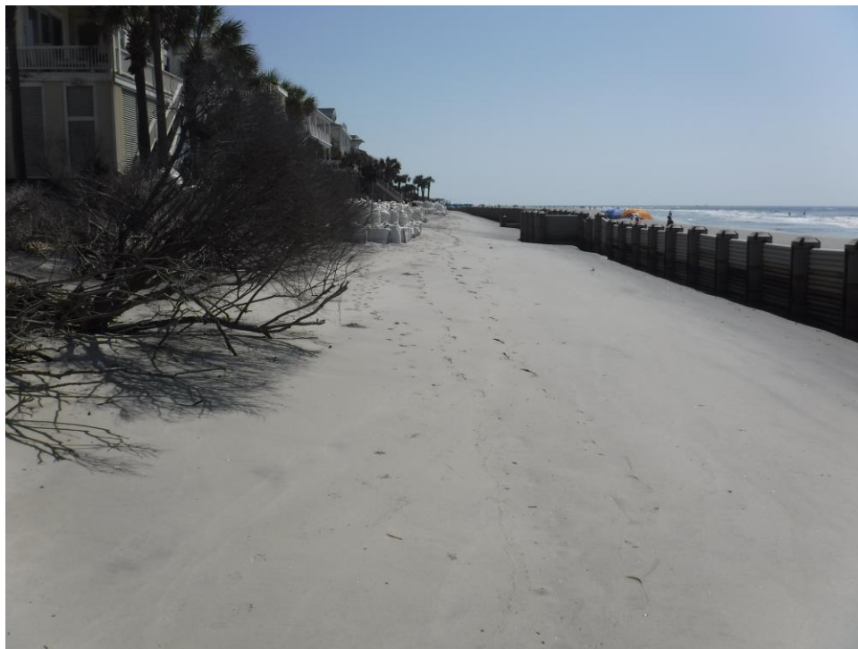
Figure 4-41. July 13 photograph from south end of WDS towards northeast
