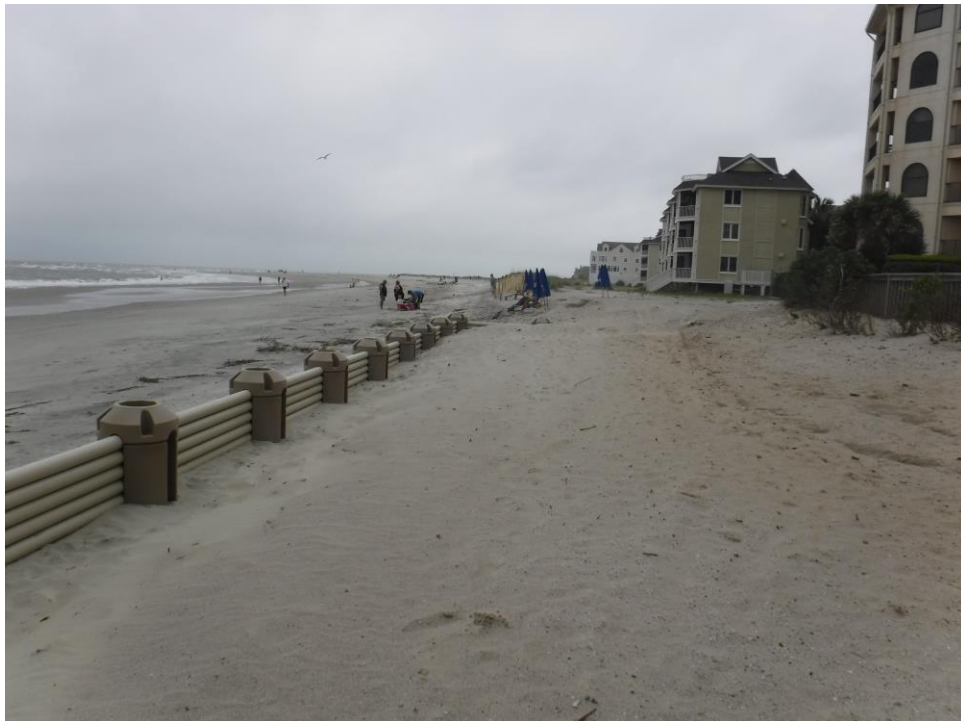
Figure 4-63. May 20 photograph looking past the west end of the WDS
