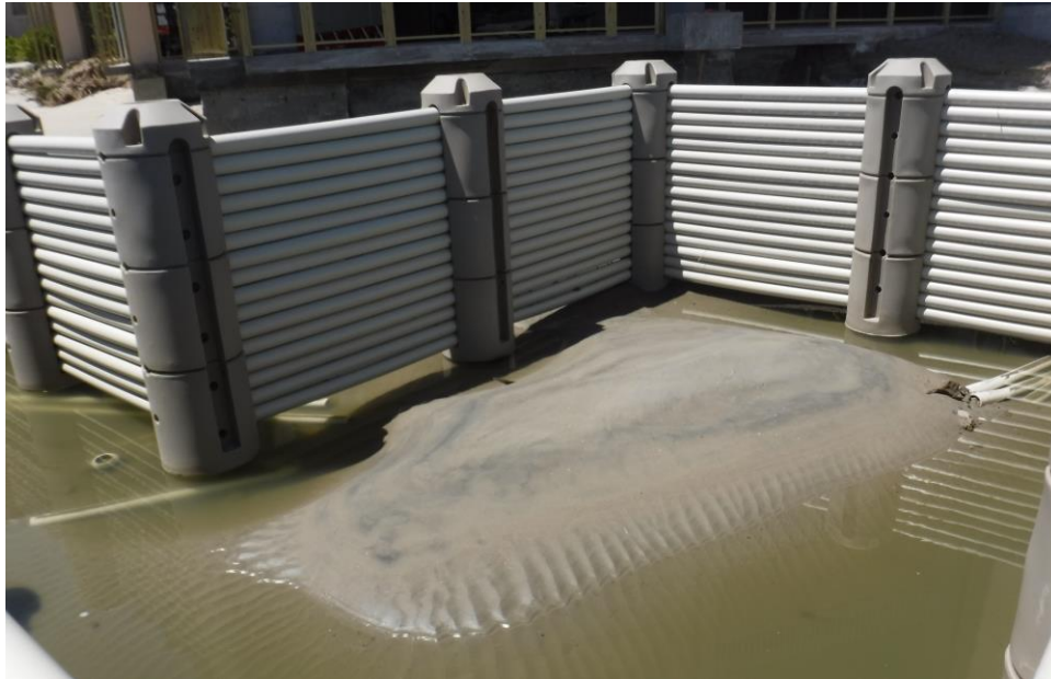
Figure 4-111. Pipes beneath WDS at Ocean Club (April 18, 2016)
