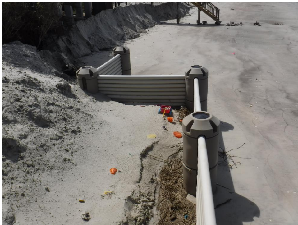
Figure 4-28. April 19 photograph looking northwest from lot 56
