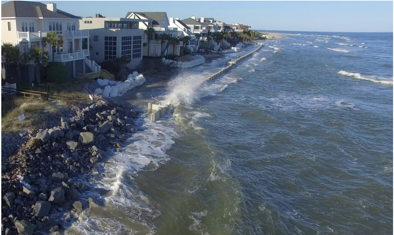
Figure 4-107. Aerial view of breaking wave at west end of BE
