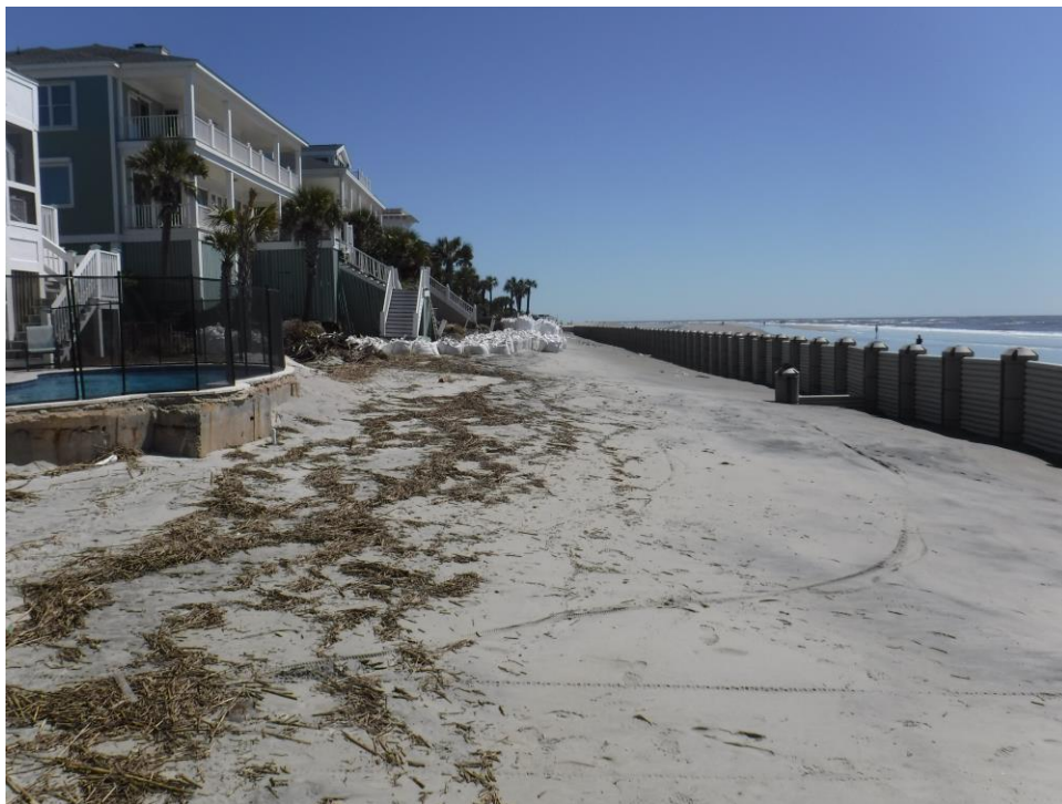
Figure 4-43. April 18 photograph from the community access point looking northeast
