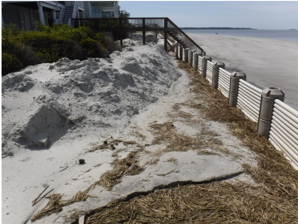
Figure 4-24. April 19 photograph looking northwest toward lot 56
