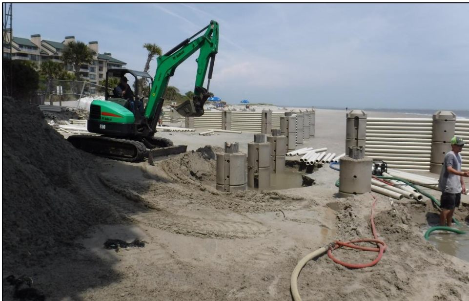
Figure 4-73. Compact excavator used for WDS installation
