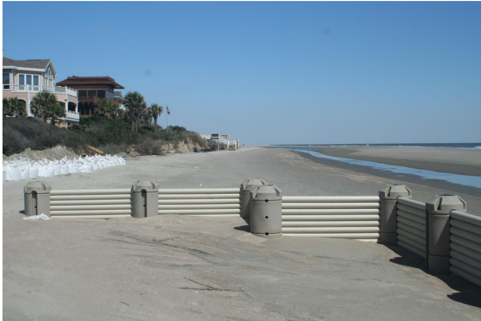
Figure 4-50. March 20 photograph from east end of WDS looking northeast
