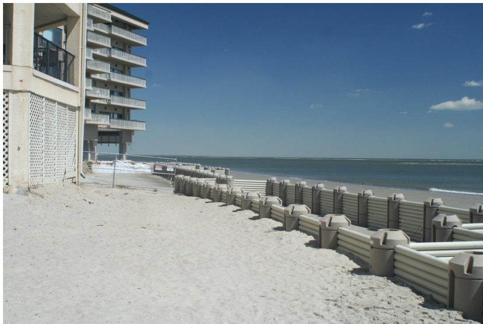
Figure 4-65. March 24 photograph looking east from SV
