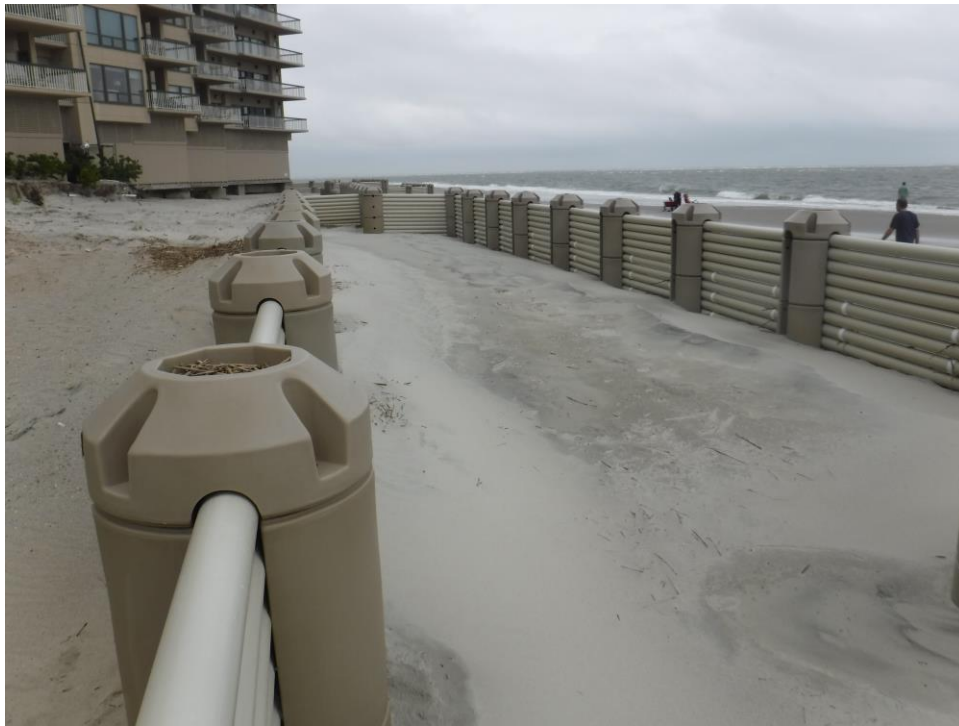
Figure 4-100. Beach without scour seaward tier of the SV WDS (May 20, 2016)
