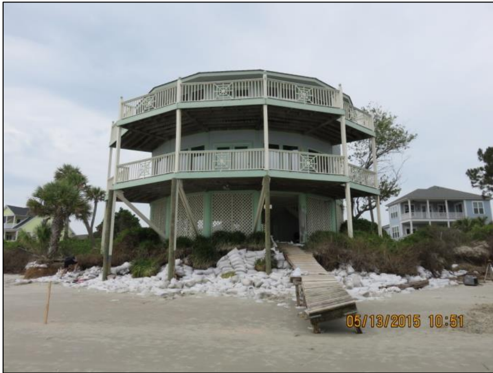
Figure 2-9. Shoreline conditions at lot 49 prior to WDS installation
