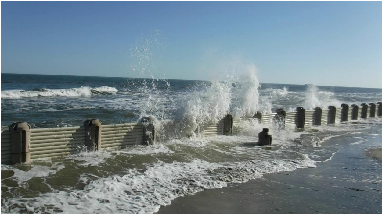
Figure 4-109. Example of overtopping at BE
