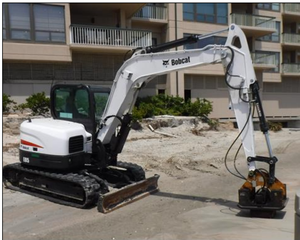
Figure 1-2. Compact excavator with vibratory driver attachment used for WDS installation
