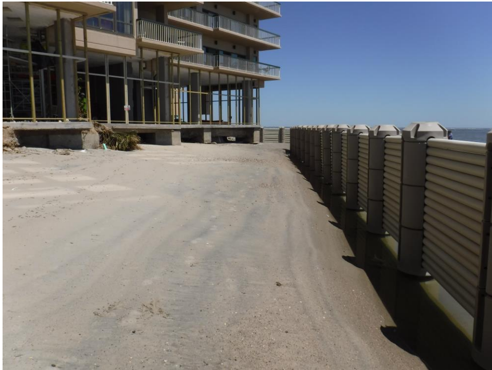
Figure 4-70. April 18 photograph looking east toward OC building
