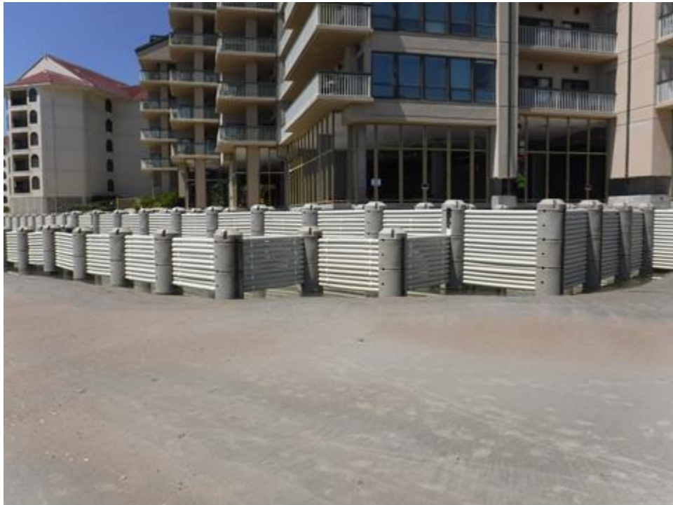
Figure 4-83. April 18 photograph of southeast corner of three-tier WDS section
