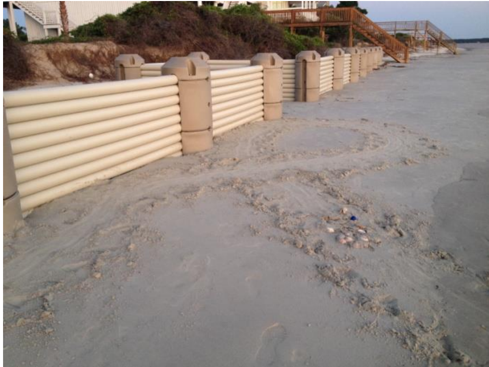
Figure 4-114. June 12, 2015 false crawl at Harbor Island (source: SCDHEC-OCRM)
