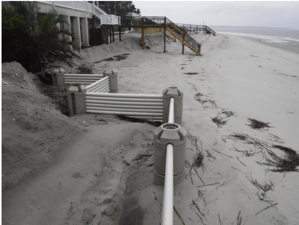
Figure 4-29. May 19 photograph looking northwest from lot 56
