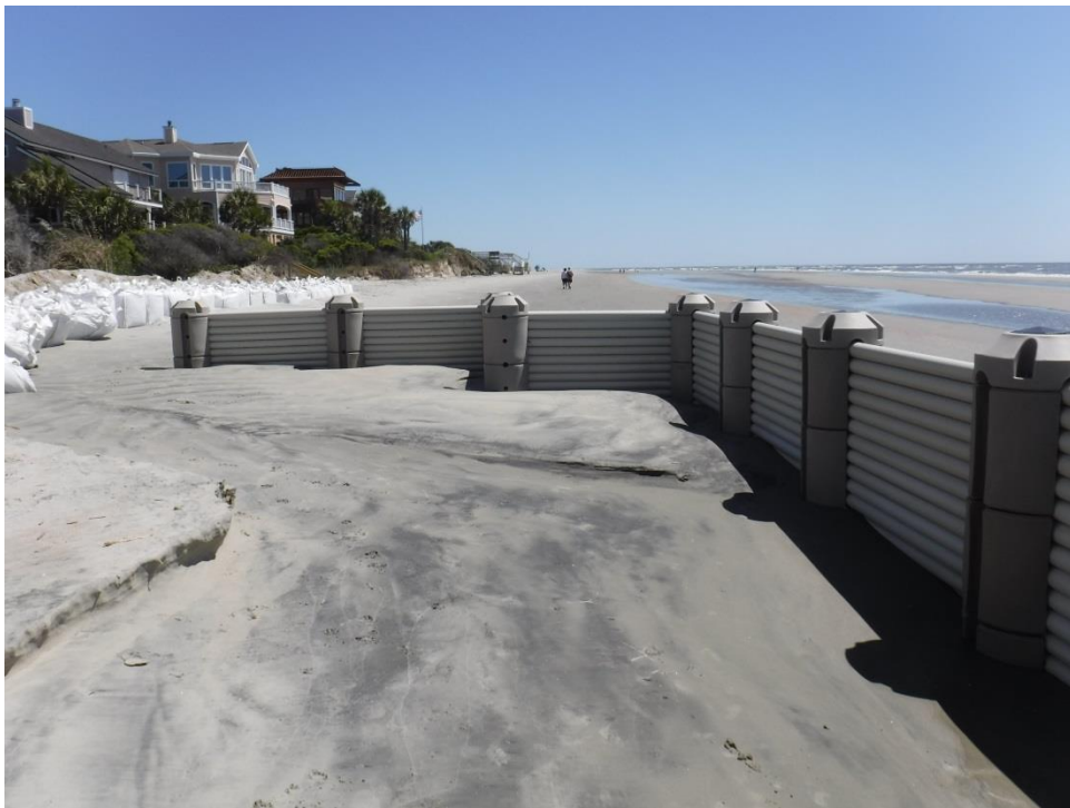
Figure 4-51. April 18 photograph from east end of WDS looking northeast
