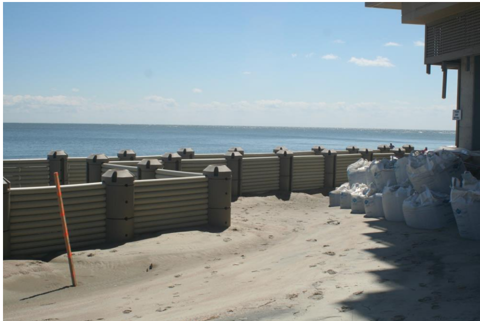
Figure 4-74. March 24 photograph from east side of OC looking south
