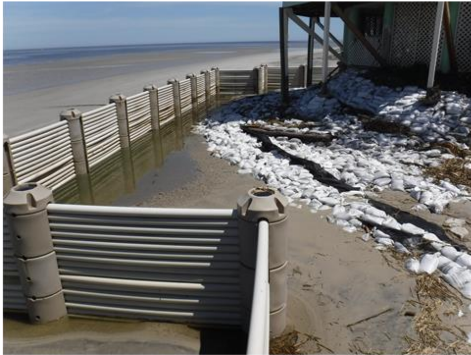
Figure 4-12. April 19 photograph looking southeast in front of lot 49
