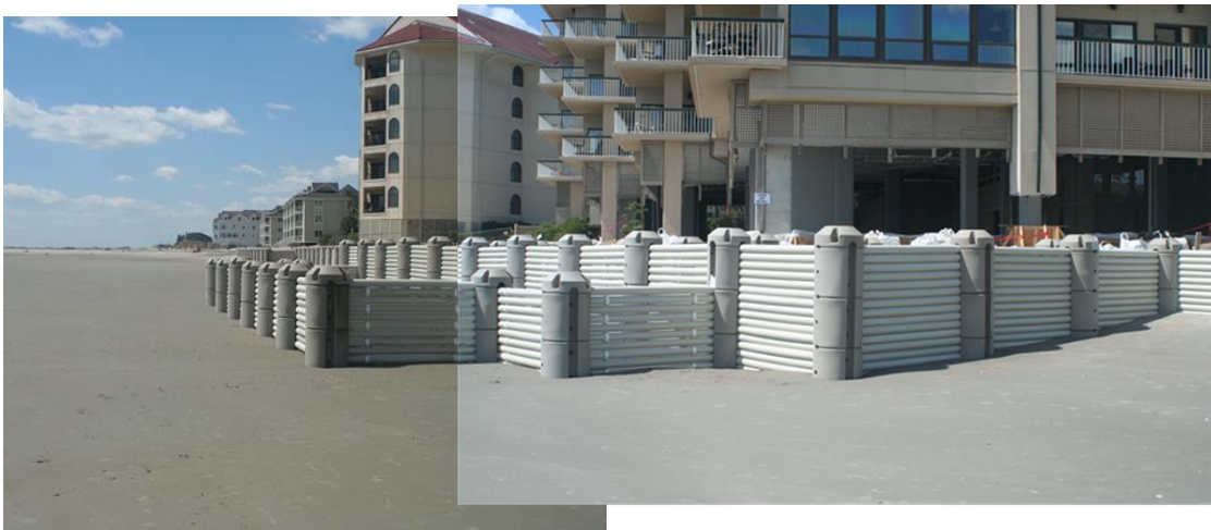
Figure 4-82. March 20 photographs of southeast corner of three-tier WDS section
