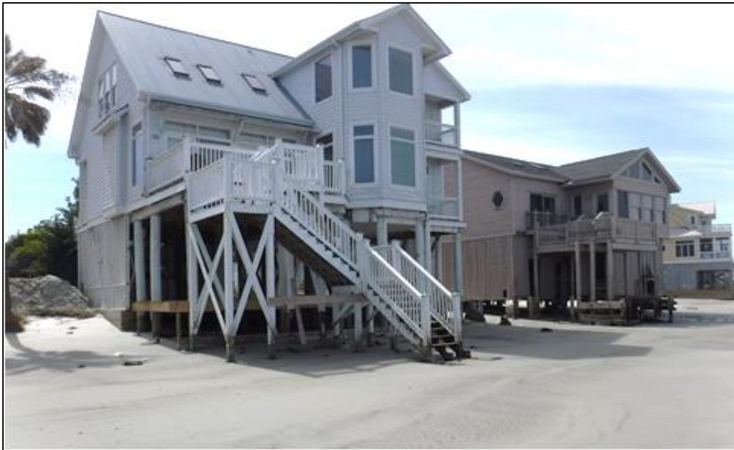
Figure 2-6. Residences undermined by erosion (April 19, 2016)
