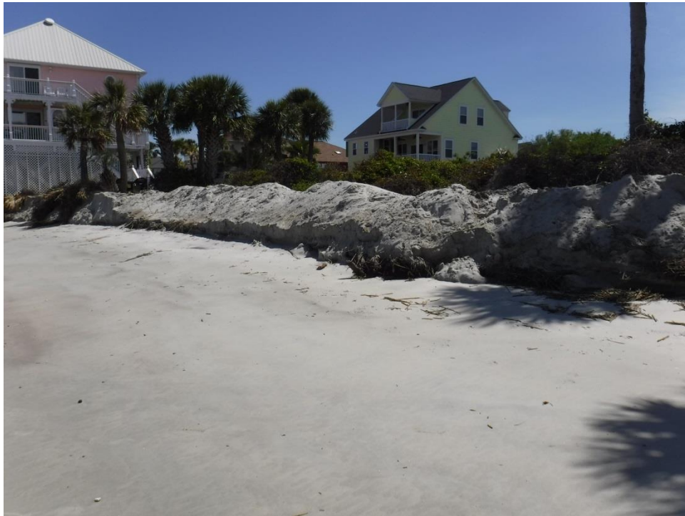
Figure 4-8. April 19 photograph of shoreline adjacent to east end of WDS
