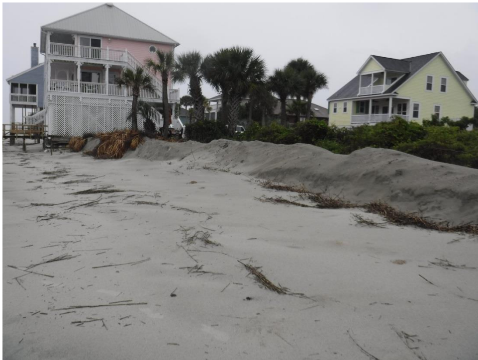
Figure 4-9. May 19 photograph of shoreline adjacent to east end of WDS
