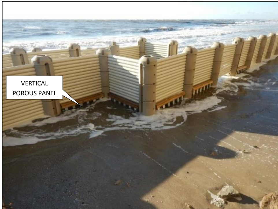
Figure 2-23. Vertical porous panels installed beneath horizontal WDS members at Ocean Club (source: SCDHEC-OCRM)
