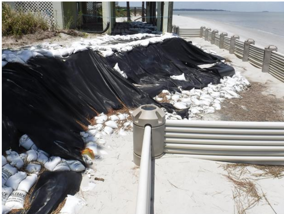
Figure 4-18. July 14 photograph looking northwest in front of lot 52
