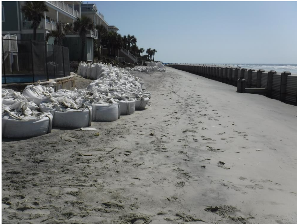
Figure 4-45. July 13 photograph from the community access point looking northeast
