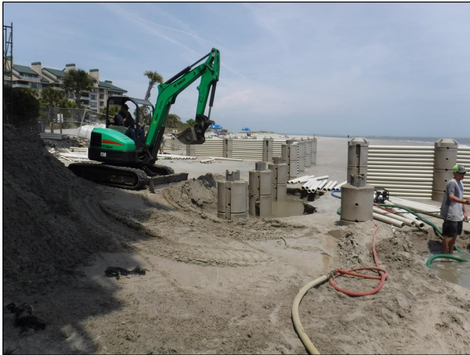
Figure 1-3. Compact excavator used for WDS installation
