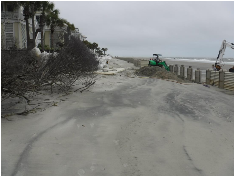
Figure 4-40. May 20 photograph from south end of WDS towards northeast
