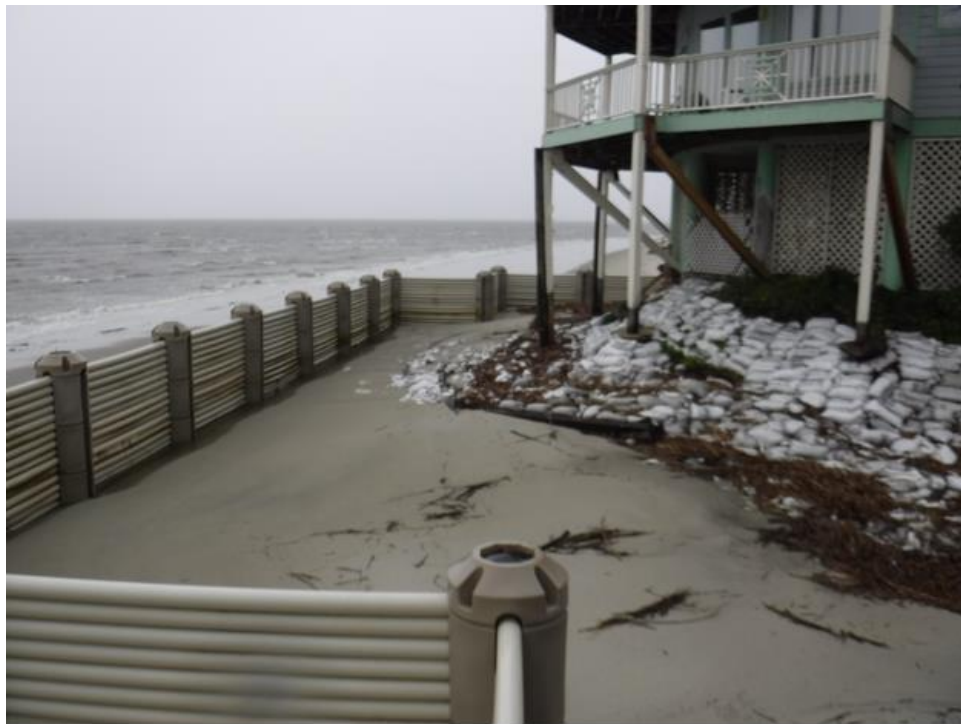
Figure 4-13. May 19 photograph looking southeast in front of lot 49
