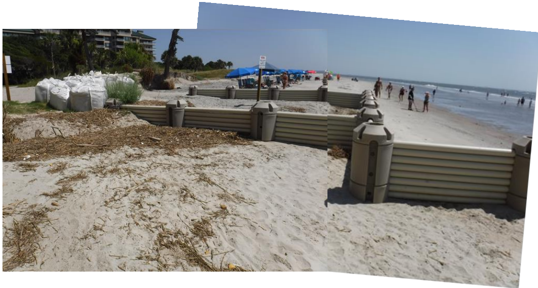
Figure 4-81. July 13 photographs from east side of OC looking east
