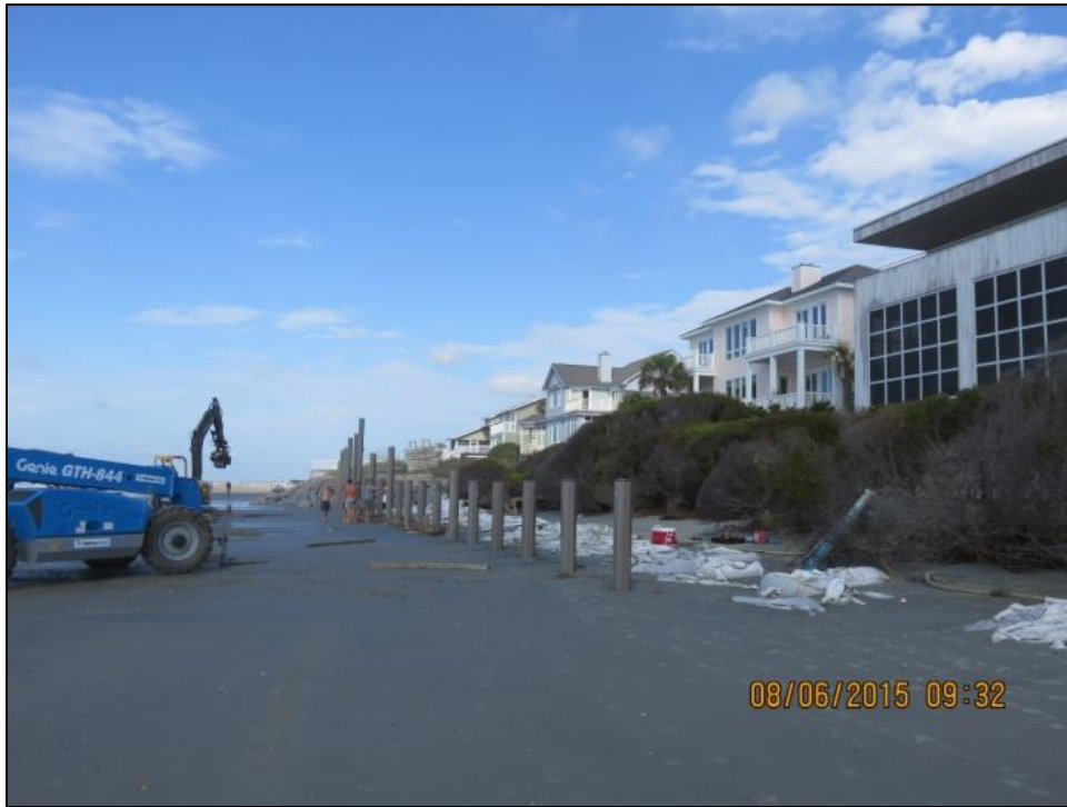
Figure 2-28. WDS at Beachwood East during August 2015 installation (source: SCDHEC-OCRM)
